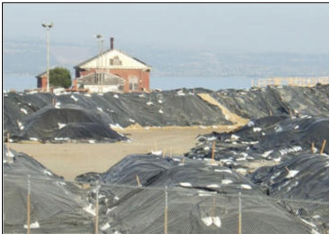
At the former naval shipyard at Hunters Point, cleanup efforts this year involved excavating 25,000 cubic yards of pipes and soil that had to be scanned for radiological residues. Photo by Arthur O'Donnell.
