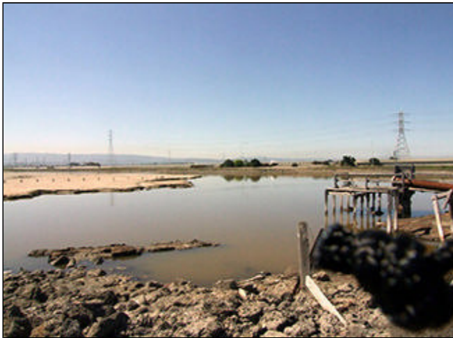
An area along the bay, now described as a "moonscape" by federal officials, will be part of a 50-year wetlands restoration effort. Initial projects will involve breaching levees, repairing water flow control facilities, and installing view points, trails and other amenities. Photo by Arthur O'Donnell.
