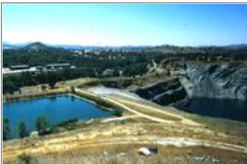
The Jamestown mine in California had a poorly designed embankment and pit liner that failed to prevent contaminated seepage into groundwater. Photo courtesy of Earthworks.
