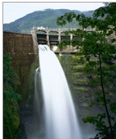
Glines Canyon Dam, a 210-foot high concrete barrier, represents the most significant dam removal project in the United States, which will begin in 2009, opening a 70-mile stretch of the Elwha River in the Olympic National Park. Photo courtesy of American Rivers.
