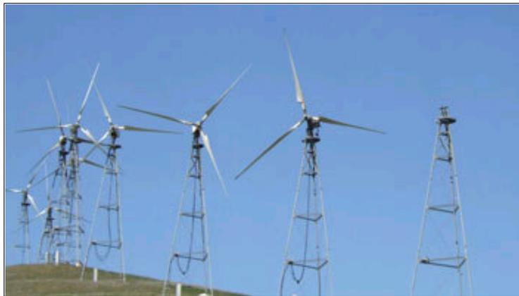
Turbines located at the end of an array of towers pose greater risk to hunting birds, so operators have been removing blades and generator boxes on hundreds of towers. Also, many older style, latticed towers -- where birds perch while hunting -- are being replaced by solid poles. Photo by Arthur O'Donnell.
